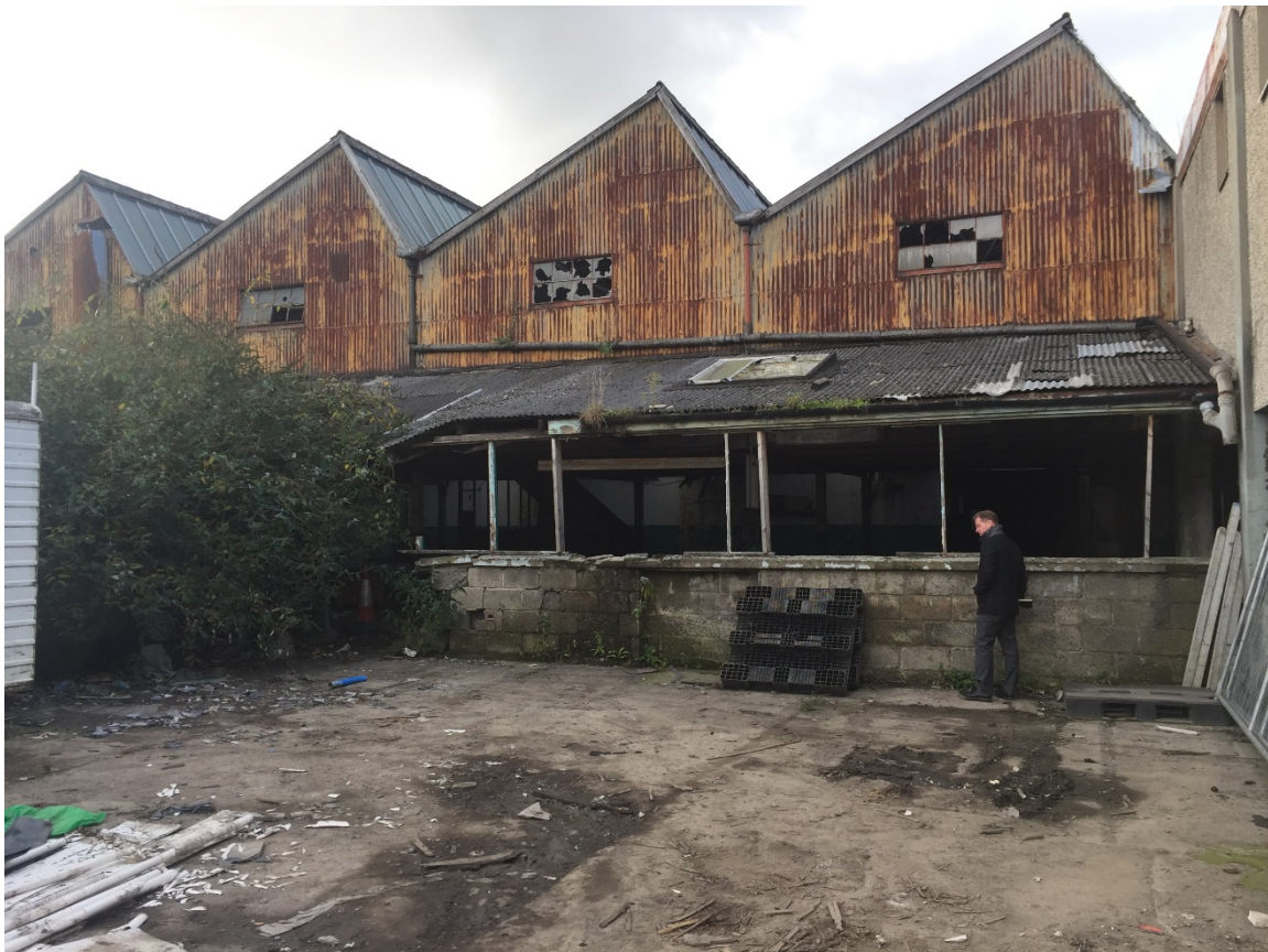
Figure 4.3 – Building F - East Elevation
